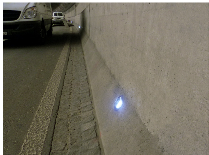
Tunnel Stephanshorn St. Gallen
